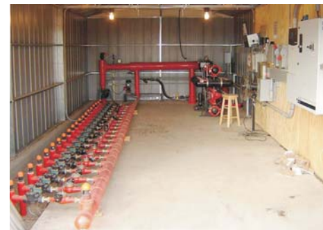
The SDI control unit includes: irrigation controller, variable speed controller, water and fertilizer flowmeters, chemical injection pump, along with numerous filters and valves.
