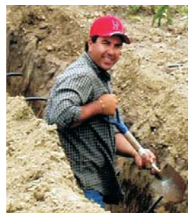
Dr. Irmak connects individual drip lines to the main lines. A total of 344 drip lines were connected.
